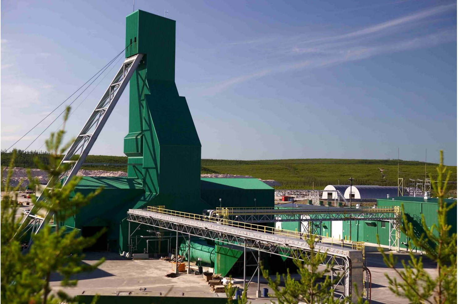
Cameco's McArthur River uranium mine in Saskatchewan.
